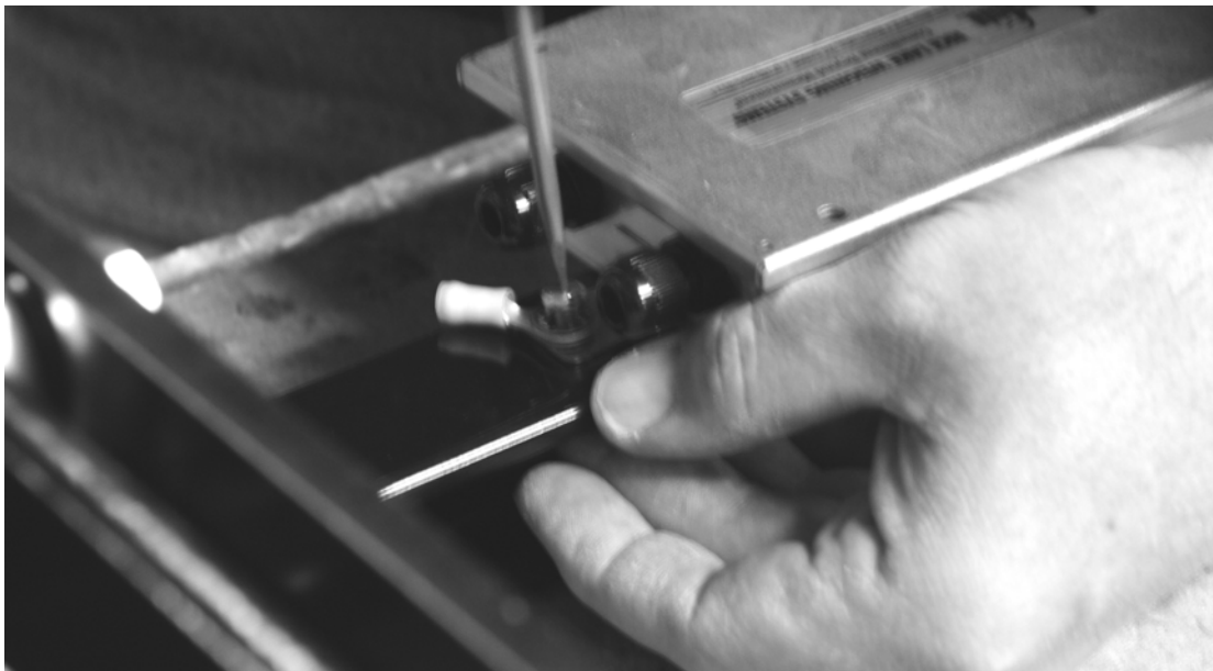
Figure 2-5. Attach the Ground Lug onto the Junction Box
